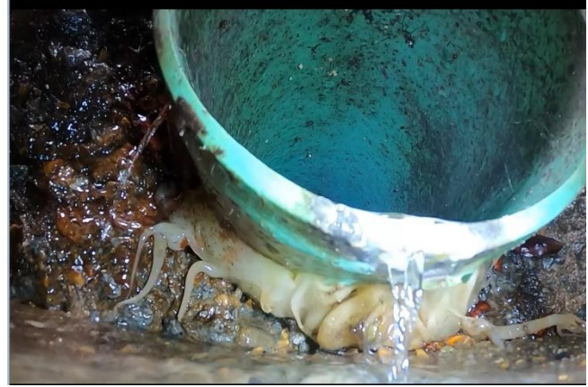
Defective Pipe Seal
